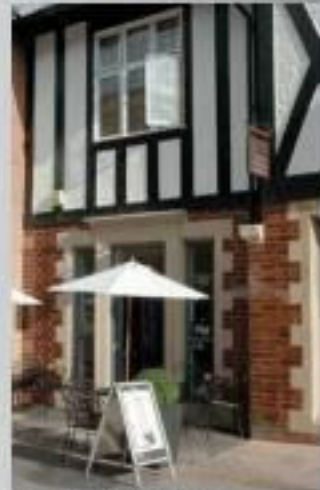
Former Barley Mow Public House
